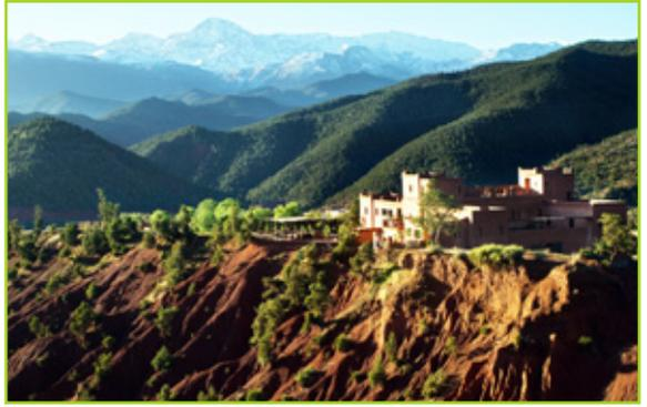
The Kasbah is one of the most eco-friendly buildings in Morocco. Constructed principally from pisé (*rammed earth*), the traditional Berber building technique, it blends easily with rock and earth around it. Thick walls provide natural insulation in the heat and along with solar panels ensure a balanced temperature. All water at the Kasbah is recycled and used in the garden and an innovative biodigester system is used to produce electricity and also compost for the fully organic garden.
